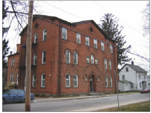
Cornwall School District #4 (rear and front), Idlewild Avenue, 1868 and 1898
