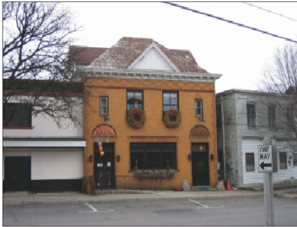
Cornwall Bank (former Village Office), River Avenue, 1897
