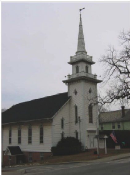
Cornwall Presbyterian Church, Hudson Street, 1856
